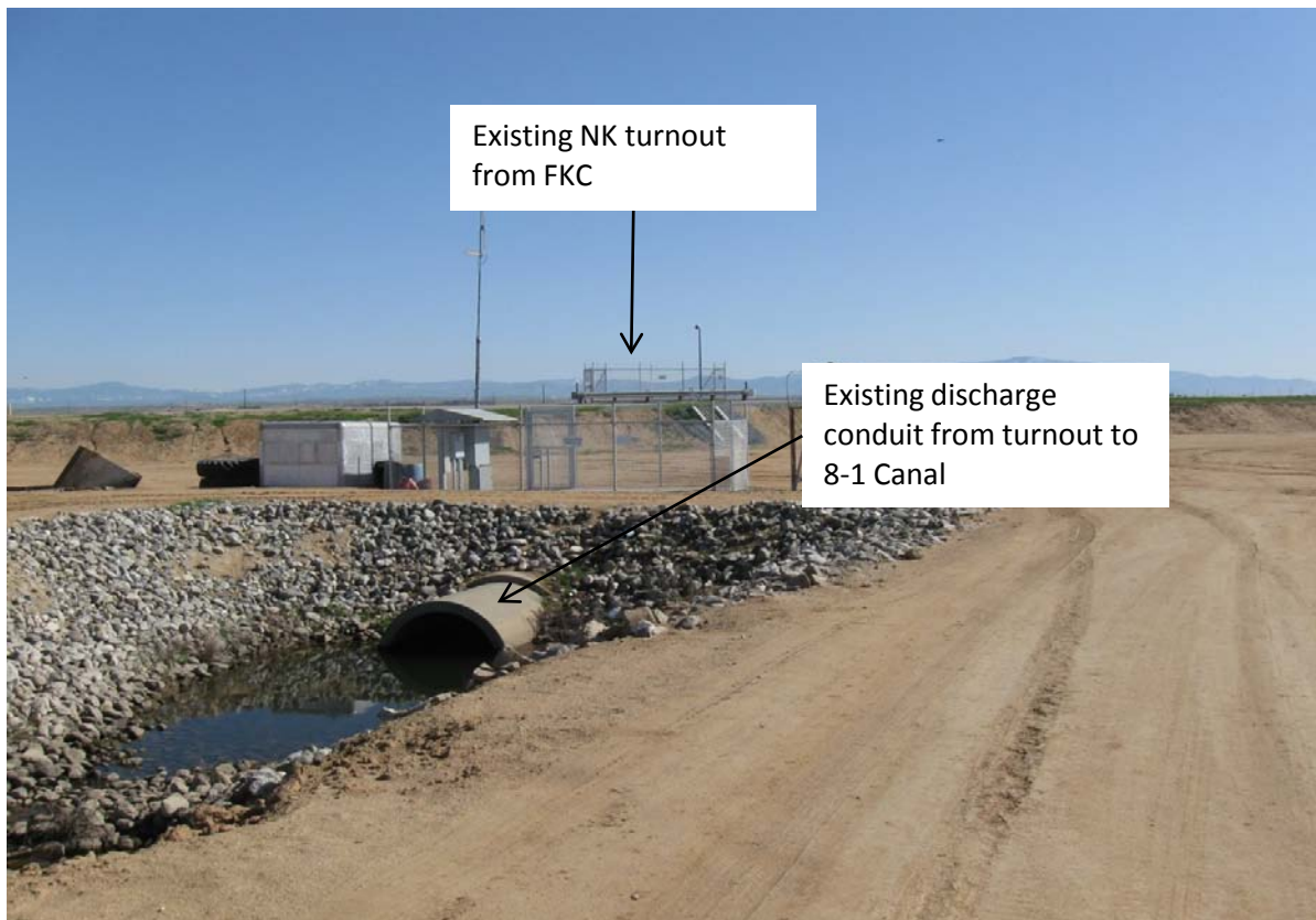
Photo 1 - Looking easterly toward the existing NK turnout from the Friant-Kern Canal
