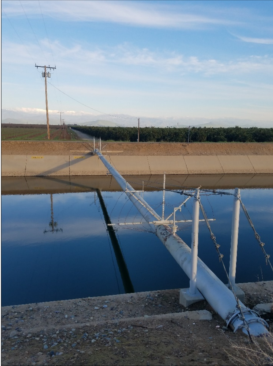
Figure 1-16. Pipeline Overcrossing on FKCs
