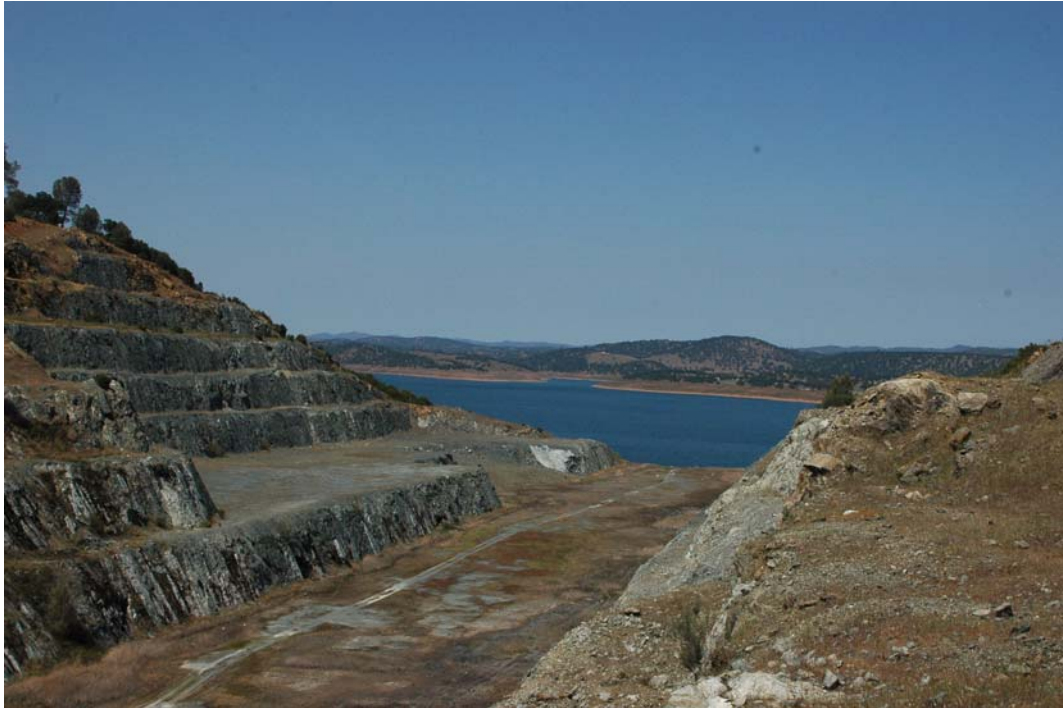
Photograph 19. New Melones Dam Spillway.
