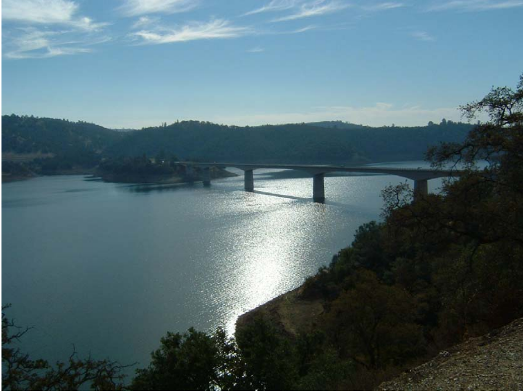
Photograph 9. View from Highway 49 Vista Point of the Highway 49 bridge and New Melones Lake.
