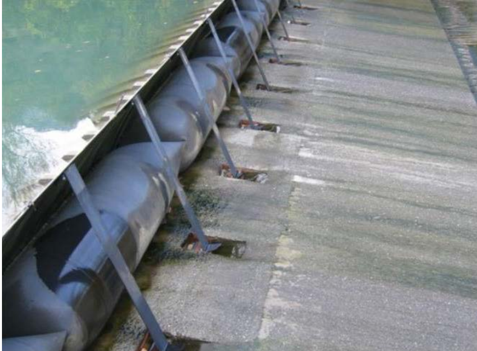
Figure 2-19. Example of Obermeyer-Style Inflatable Gates
