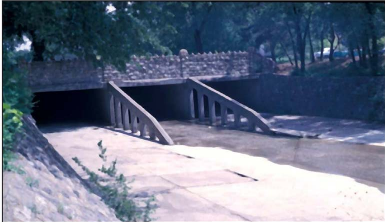
Figure 2-7. Debris Fins Incorporated at Headworks Structure (Example)
