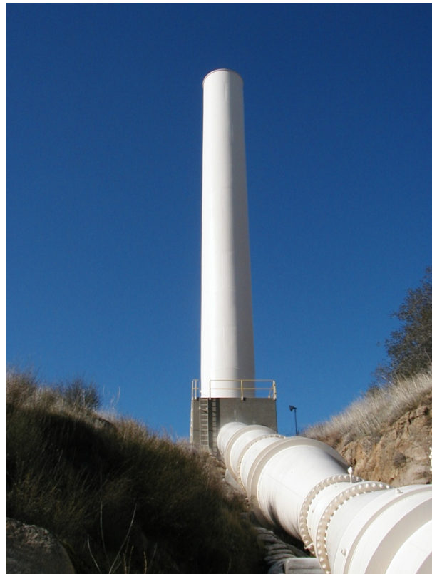
Figure 3.6-2 Existing East Surge Tower
