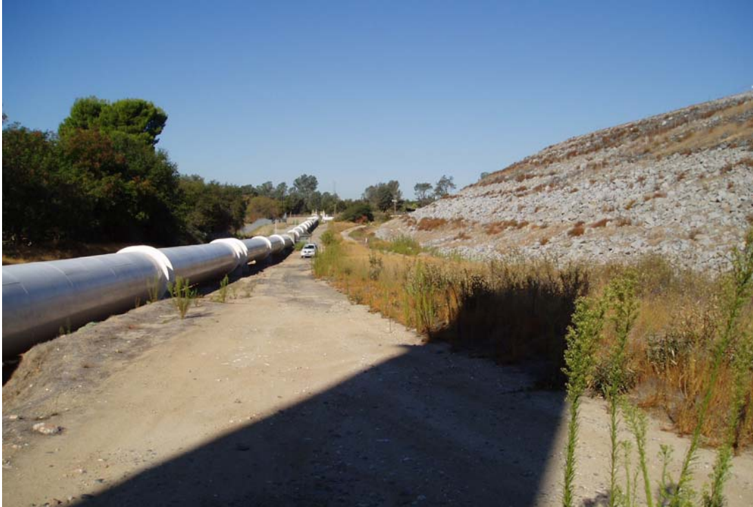
Figure 3.6-1 Existing 84-inch Raw Water Pipeline and Right Wing Dam
