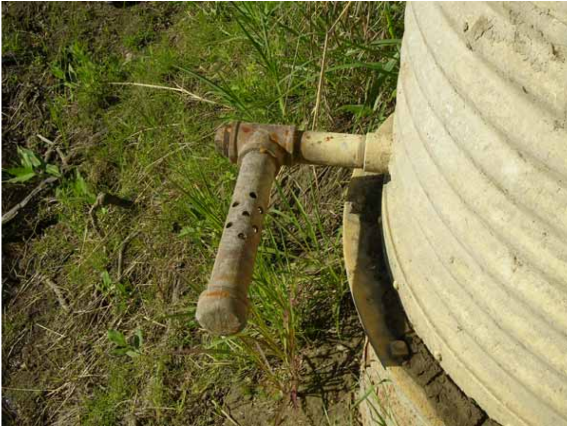
Figure 7: Two-inch diameter metal pipe protruding from the bottom of the corrugated metal housing.
