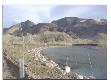
An example of completed bank stabilization along the outside of a new river meander at the McCarran Ranch Project site.
