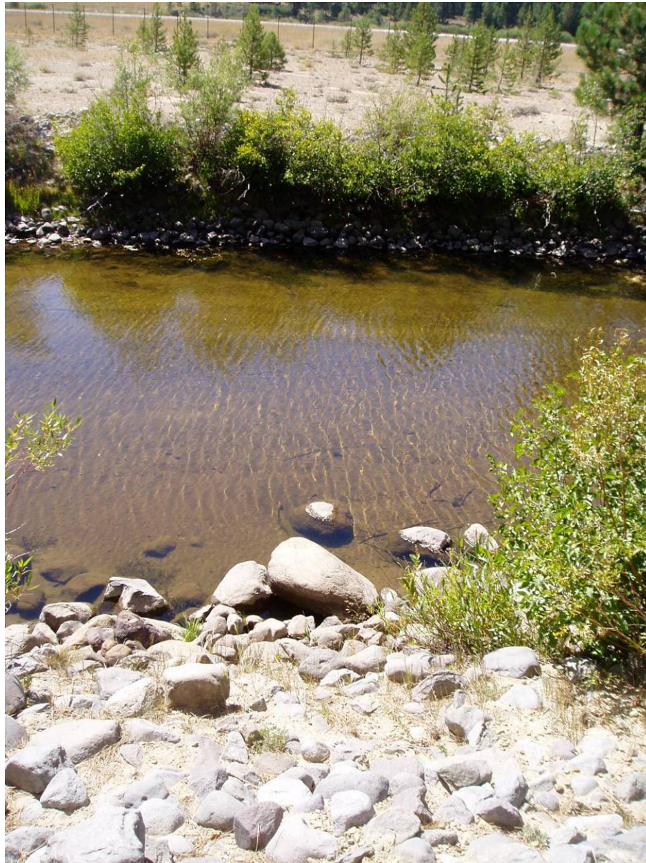
Figure 4.5-4 Cross-Sectional View of the Typical Homogeneous Trapezoidal Channel Form in the Reaches Adjacent to the Airport (Note the predominantly sand bottom and lack of cover for fish.)
