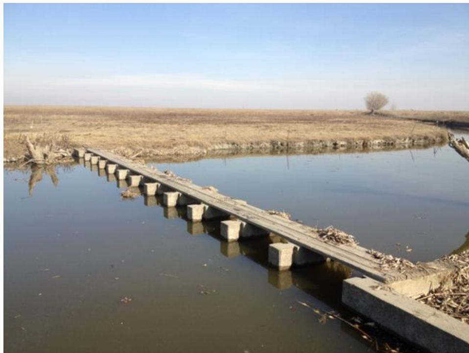
Figure 3.1-4. View of the Upper Merced Weir, Looking East
