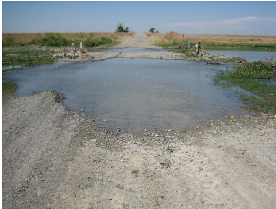
Figure 3.1-2. View of Dan McNamara Road Crossing the Eastside Bypass during Inundation, Looking North
