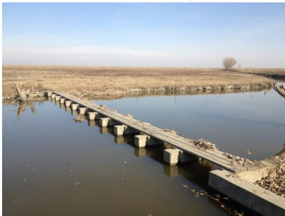
Figure 2-10. Upper Merced Weir #2 Looking East at the Right Bank
