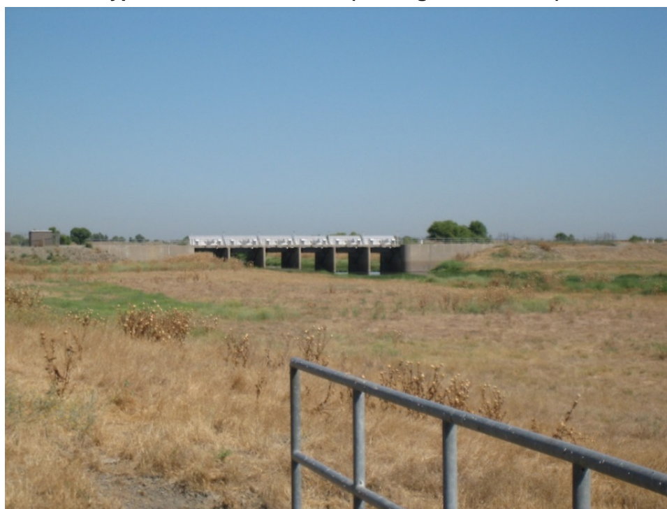
Figure 2-2. Eastside Bypass Control Structure (looking downstream)
