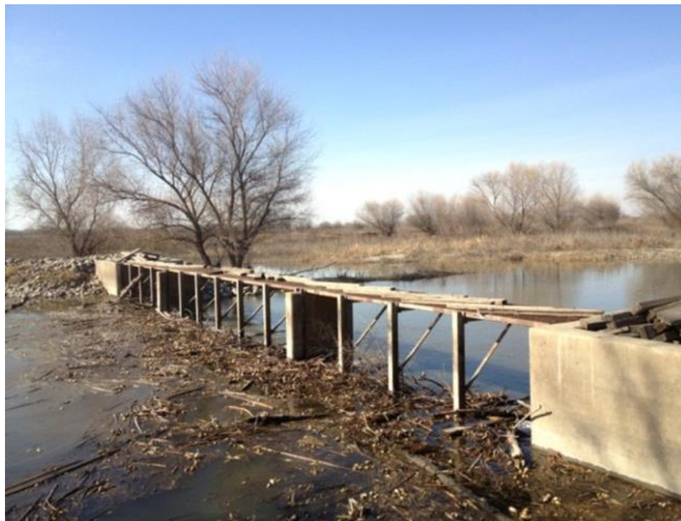
Figure 2-9. Lower Merced Weir #1 Looking Downstream
