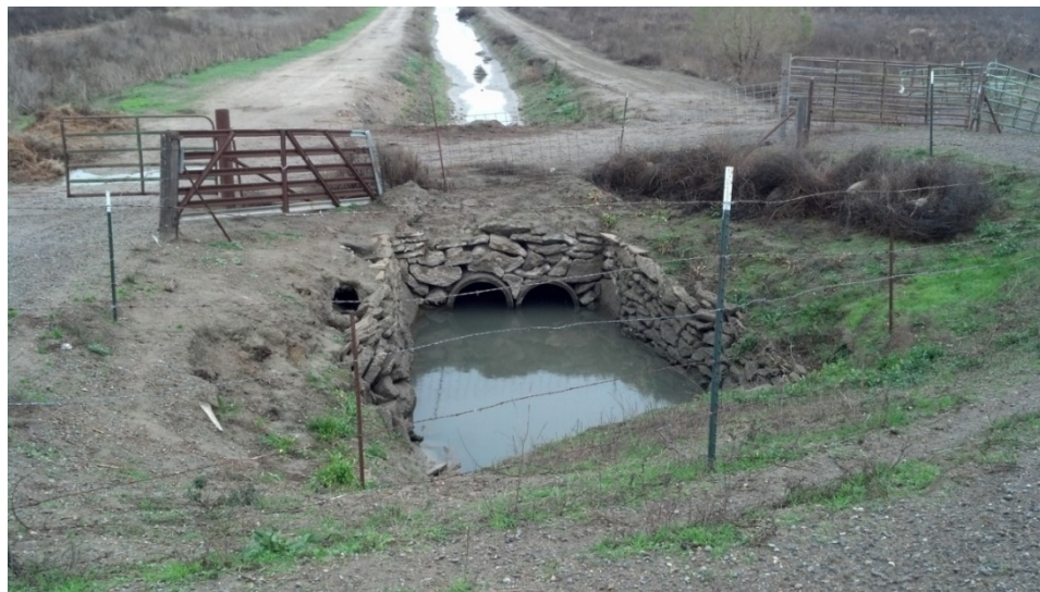
Figure 2-1. Irrigation Canal and Culvert Crossing at Existing Levee
