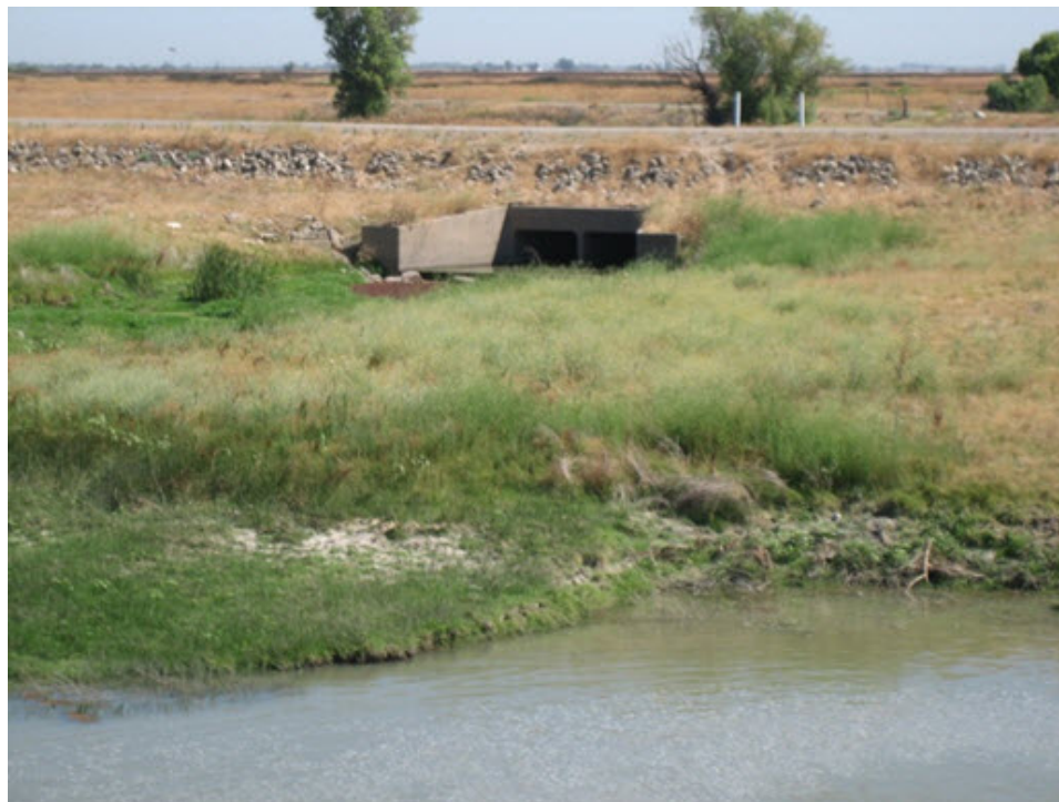
Figure 2-4. Gated Outflow Structure at Eastside Bypass Control Structure
