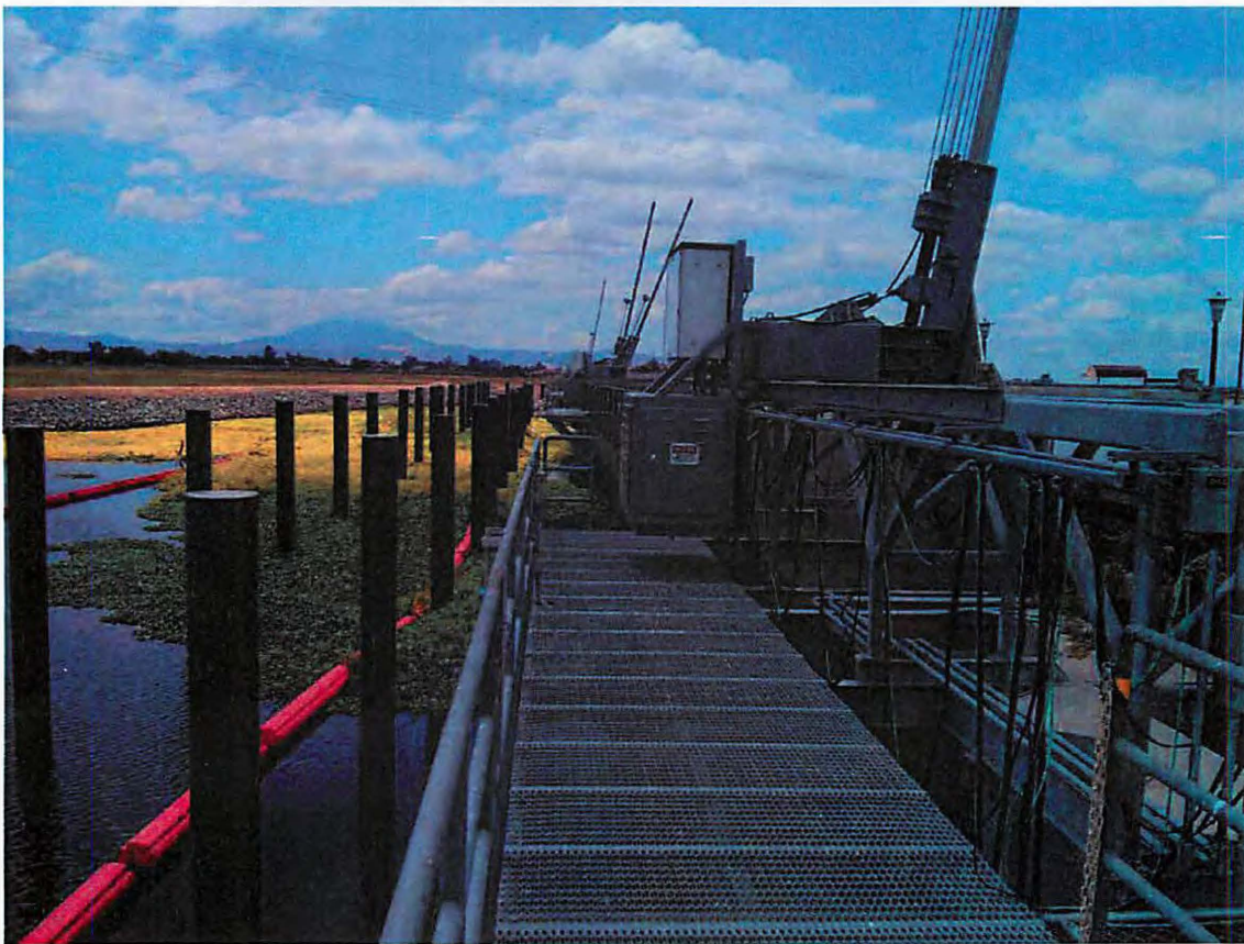
Figure 5. Existing safety deck and hydraulic rakes on the northeast side of the RSFS (Reclamation 2016).
