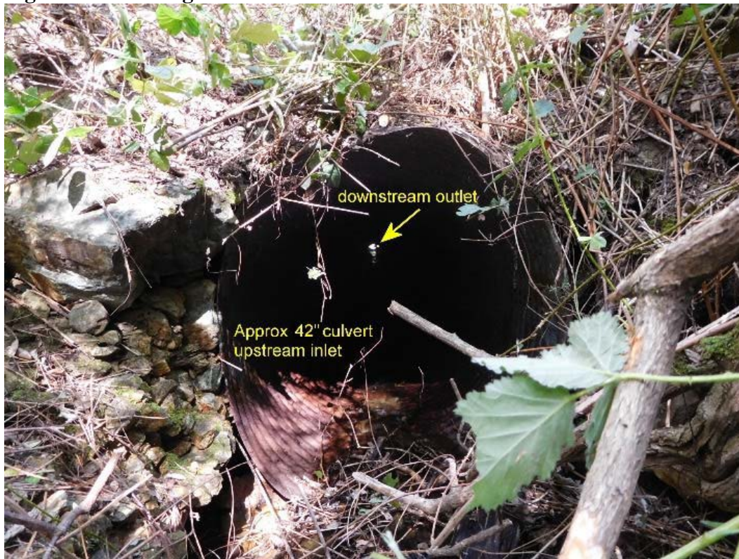
Figure 4C: Existing culvert inlet
