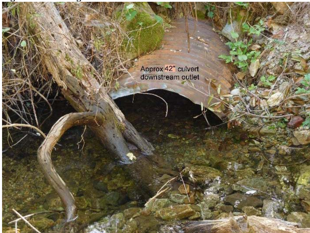
Figure 4D: Existing culvert outlet
