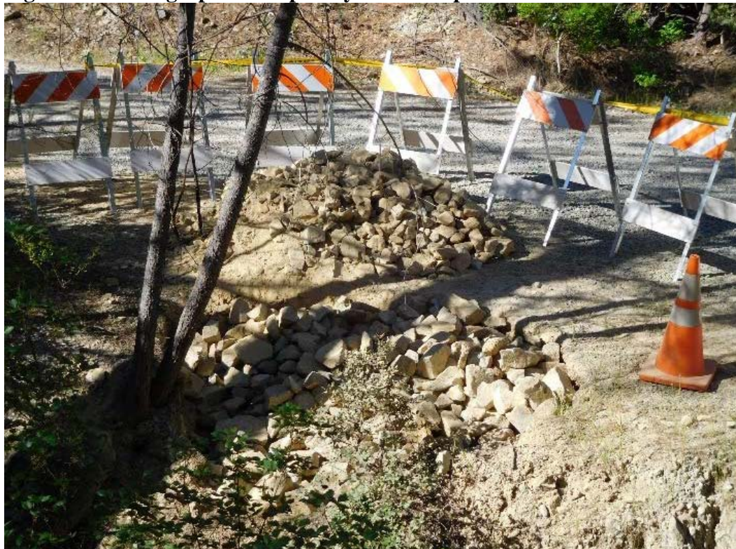
Figure 4B. Photograph of temporary culvert repair
