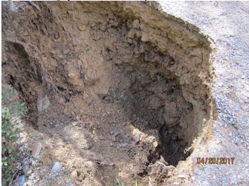
Figure 4A. Photograph of sinkhole created by failed culvert
