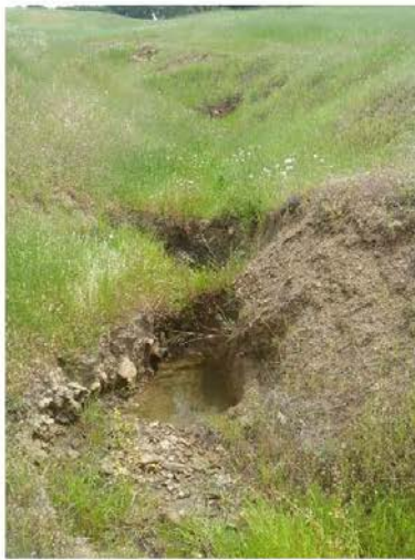
Figure 2: Pond 8 spillway erosion
