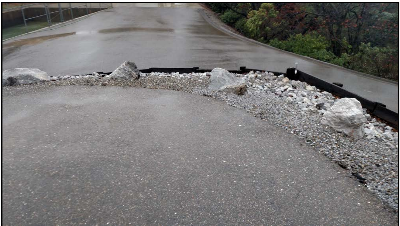
Figure 3B. Photograph of the parking lot surface behind the retaining wall to north and gravel and boulder mix to be removed prior to installation of the new retaining wall.
