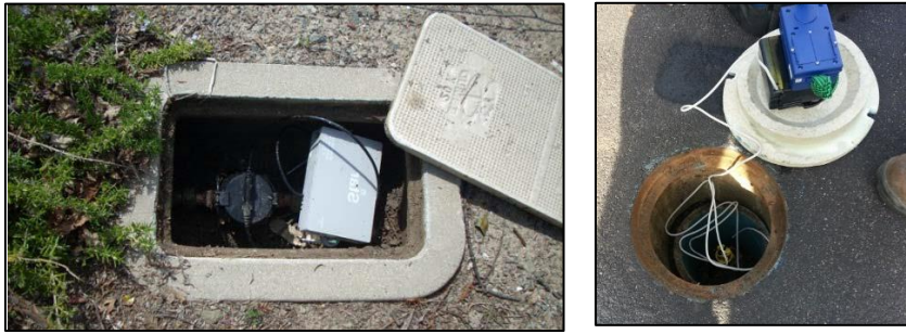
Figure 3 Example of installed meter and leak detection
