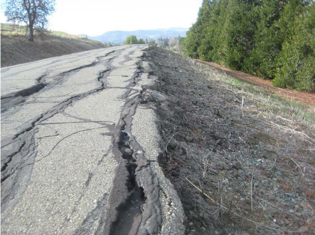
Figure 2: Longitudinal and Transverse Cracking
