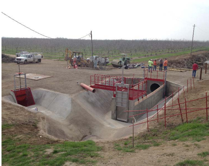
Figure 3. GHMWC Long-Crested Weir on Main Canal at Rice Canal/Orchard Ditch Heading.
