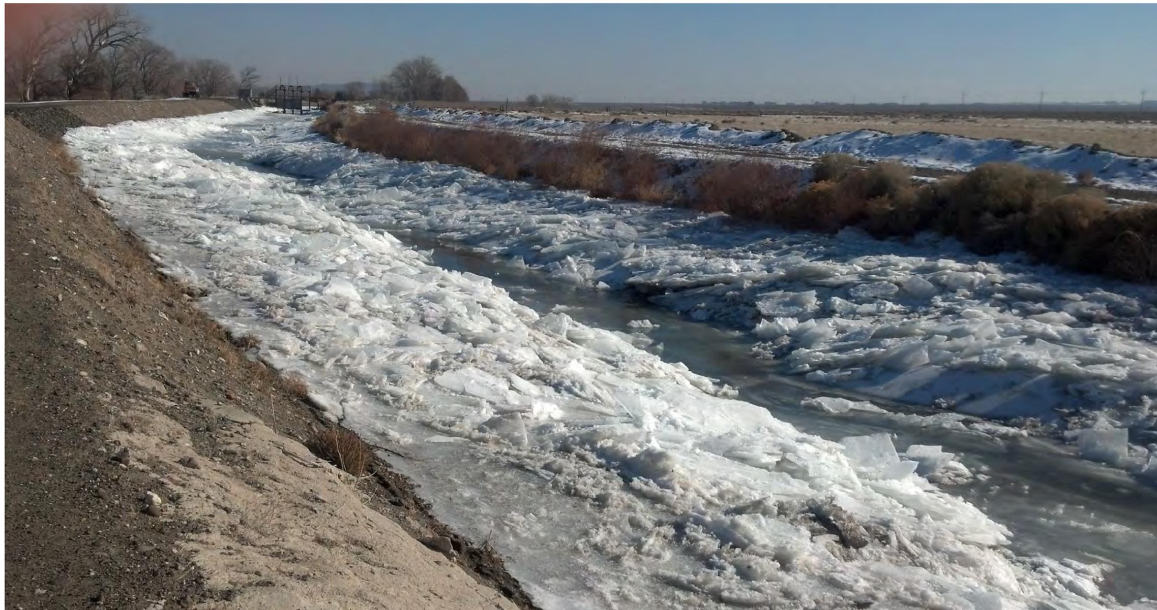
Ice buildup along the Truckee Canal. Photo credit: Truckee-Carson Irrigation District
