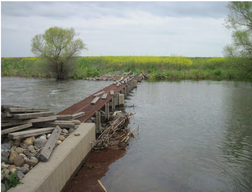
Figure 3-4. Merced National Wildlife Refuge Weir April 10, 2010. Note the two left weir bays blocked by debris.
