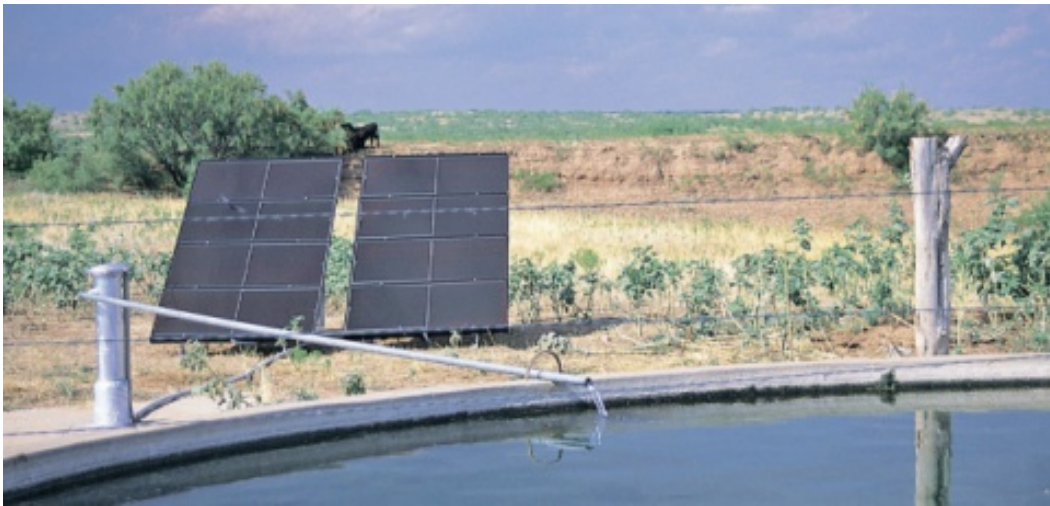
Figure 8. Example of a solar well pumping unit
