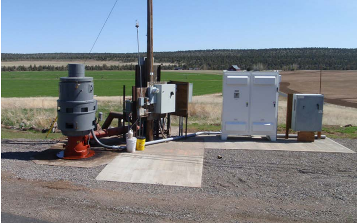
Figure 6. Example of a variable frequency drive unit on a well.
