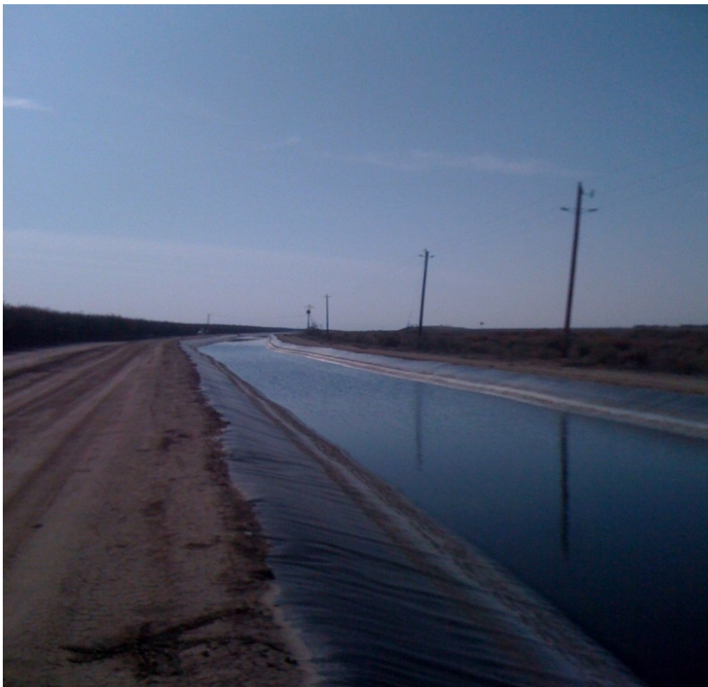
Figure 5. Example of a poly liner installed on a canal
