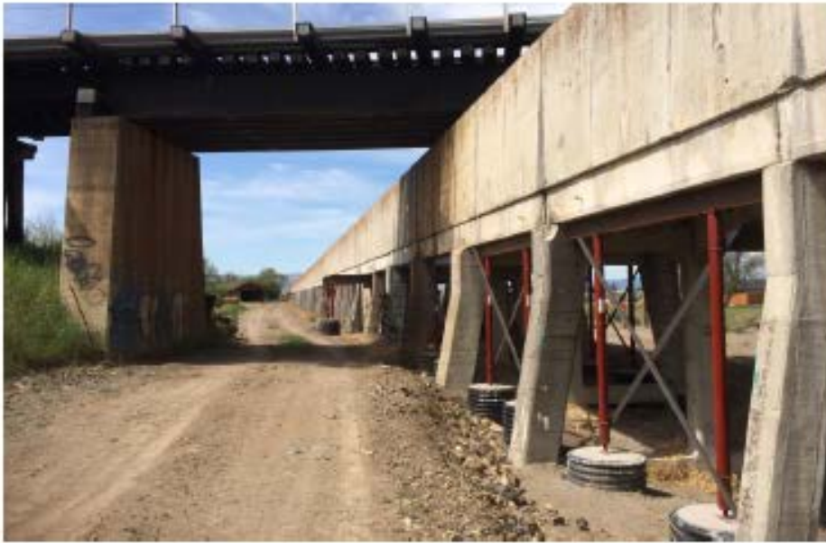
(Photo 4) C Flume crossing under the BNSF railroad
