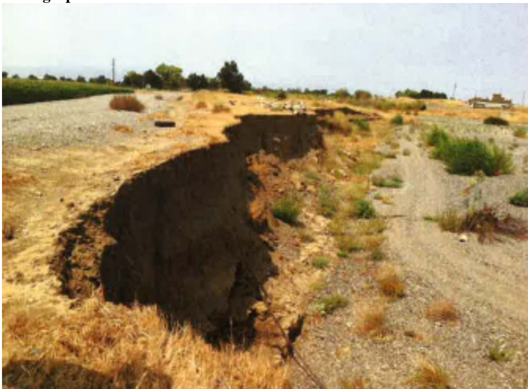
Photograph 2: View to north of bank erosion requiring material for repair.
