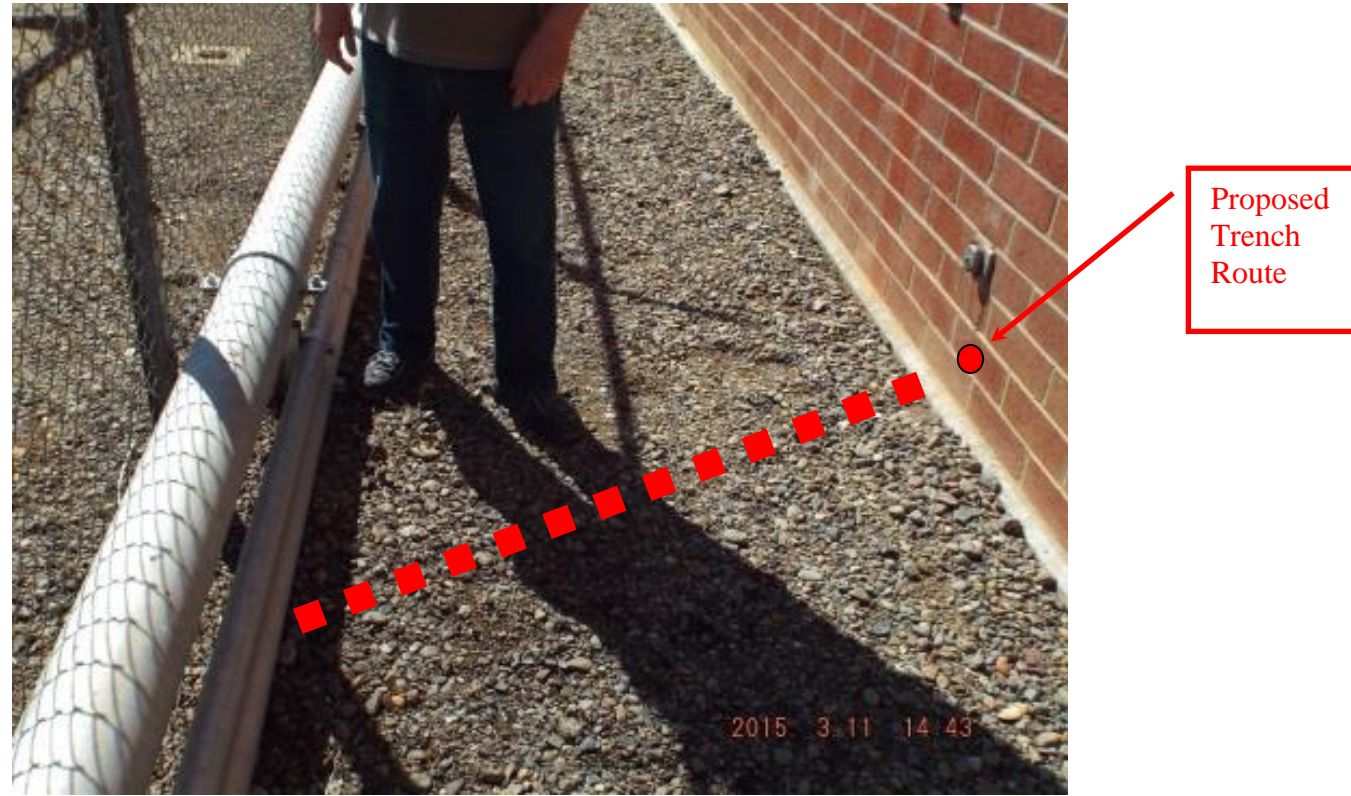
Figure 3 Proposed Trench Route at O'Neill Substation
