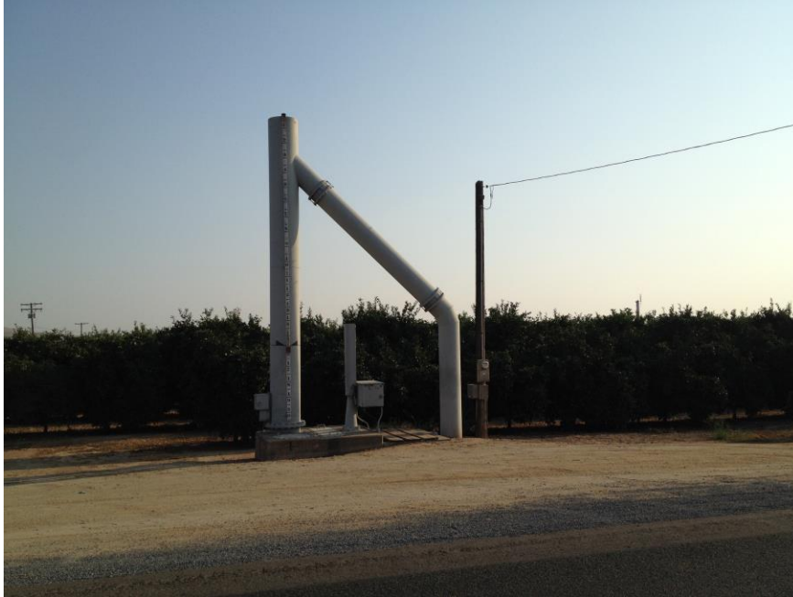
Photo 3: 68 Main Lateral – Junction Box No. 3 where SCADA equipment and above ground low-flow bypasses would be installed. Note structure as described in report. All Junction Boxes are similar in structure.
