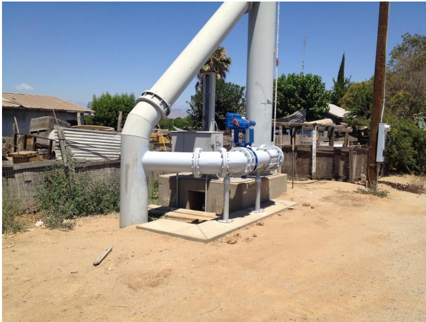
Photo 4: Typical above ground bypass as installed in 2014 as part of the District's Control System Project – 69 Main.
