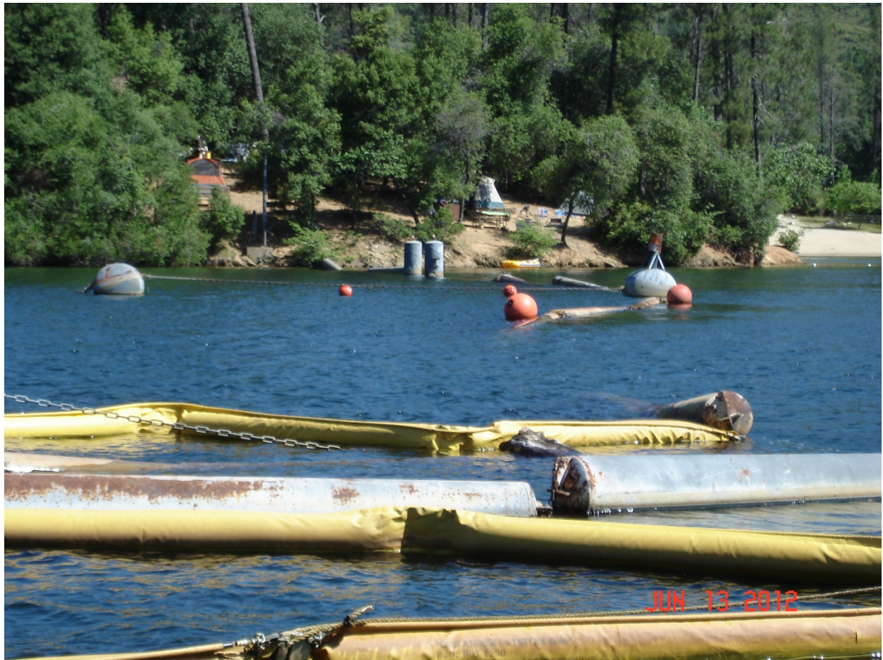
Attachment 2. Photo of the existing Oak Bottom Temperature Curtain in a dilapidated state. Note: the yellow boom is to highlight the partially sunken floatation tubes as safety hazards.
