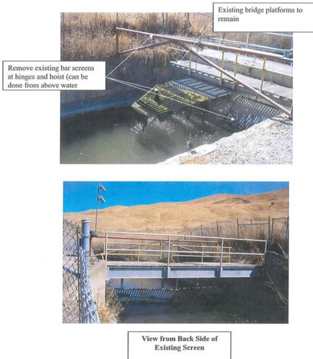
Figure 2 - Existing Bar Screen (Figure by Contra Costa WD)
