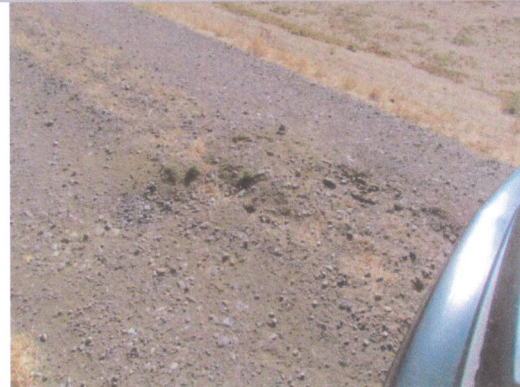
Looking north a repaired rodent hole on levee crown.
