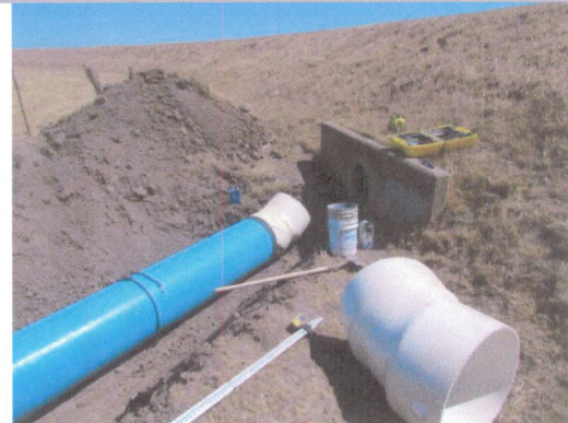
Looking east at installation of 18" pvc pipe into 24 inch drain pipe on landside slope.
