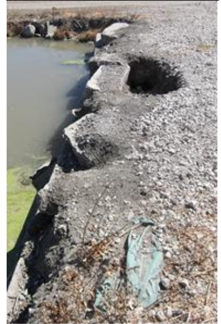
FIGURE 6: Barstow Ave. Sinkhole
