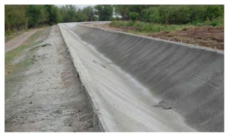
Figure 4 - Fiber-reinforced shotcrete application. Source: AW Blair Engineering (2011)
