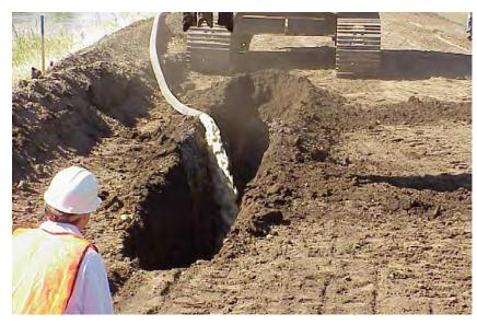
Figure 6 - Placement of slurry in prepared trench. Source: CSU Chico Research Foundation (2006)
