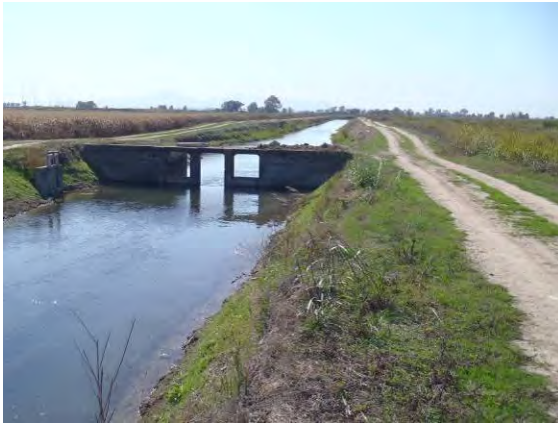
55. Lower Belding Lateral looking southwest at first check/weir west of junction with Upper Belding Lateral
