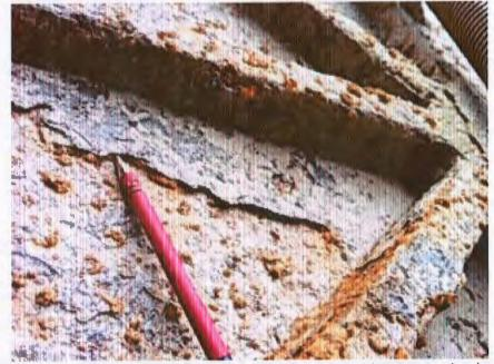
Photo 2: Upstream condition of lower gate leaf. This shows a coating system that has failed with excessive corrosion.
