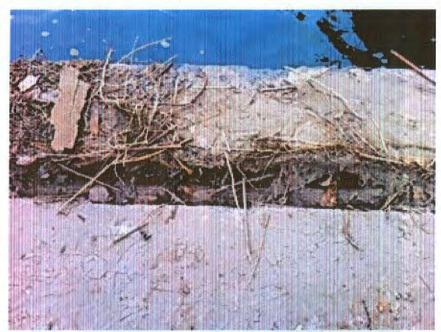
Photo 3: Typical condition of a canal gate seat embedded in the sill board. Note how seat has broken down and decayed.
