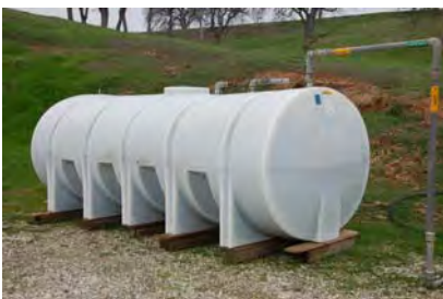
Pic #M1 Supplemental septic storage tank.JPG
