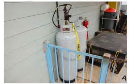
Pic #H26 Marina propane storage for unit heater.JPG
