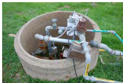
Pic #M2 Utility crossing manifold.JPG
