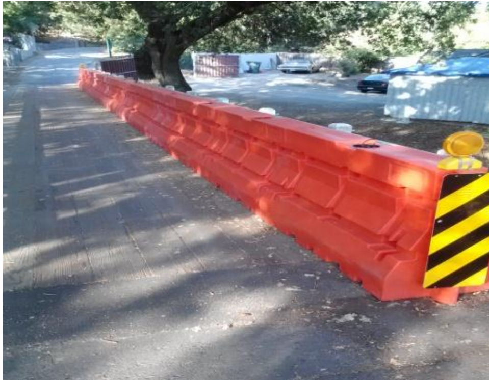
Figure 5 Barrier to Prevent Access to the Damaged Portion of the Bridge
