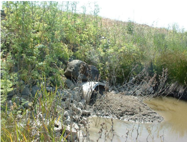
Figure 3 Sinkhole Material Extruding from Failed Culvert
