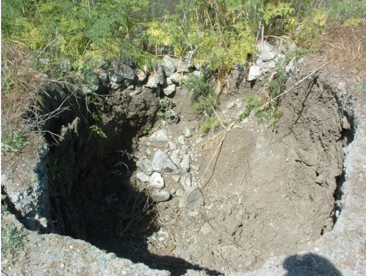
Figure 2 Levee/road Sinkhole from Collapsed Culvert
