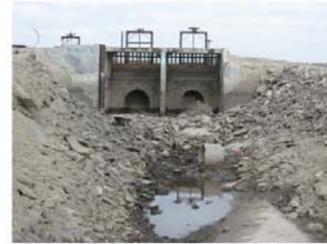
SITE #1. PACKWOOD SPILL STRUCTURE (TWO 36" GATES)
