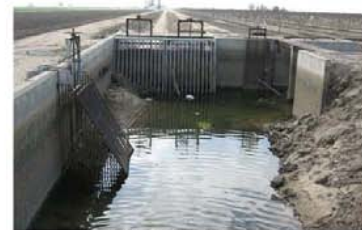
SITE #1 PACKWOOD SPILL STRUCTURE (TWO 36" GATES)
