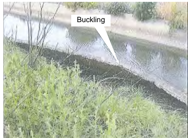
Figure 10 Liner has lifted about 2-3 feet. Note lack of vertical support (GEI 2011).
