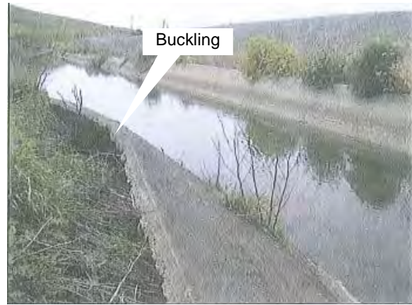
Figure 9 View of lining buckling looking downstream (GEI 2011).
