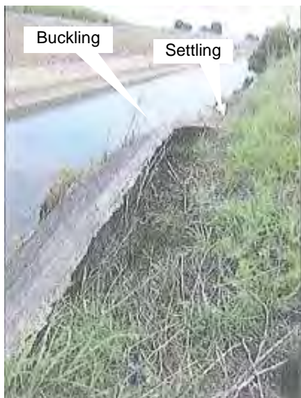
Figure 8 View of Canal lining buckle and settling looking downstream (GEI 2011).
