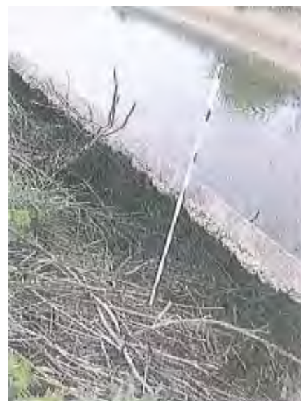
Figure 11 Close-up of Canal lining buckle with 2-3 feet of vertical displacement (GEI 2011)
