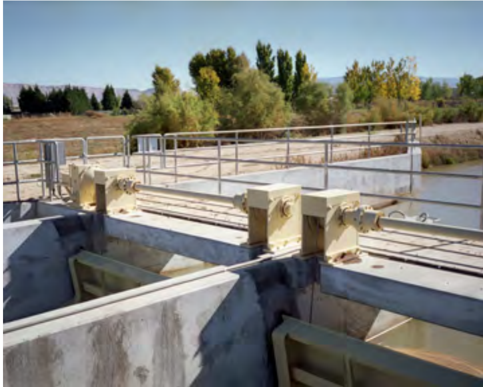
Figure 4 –Example of automated power radial gate hoist proposed for Rogers Canal
