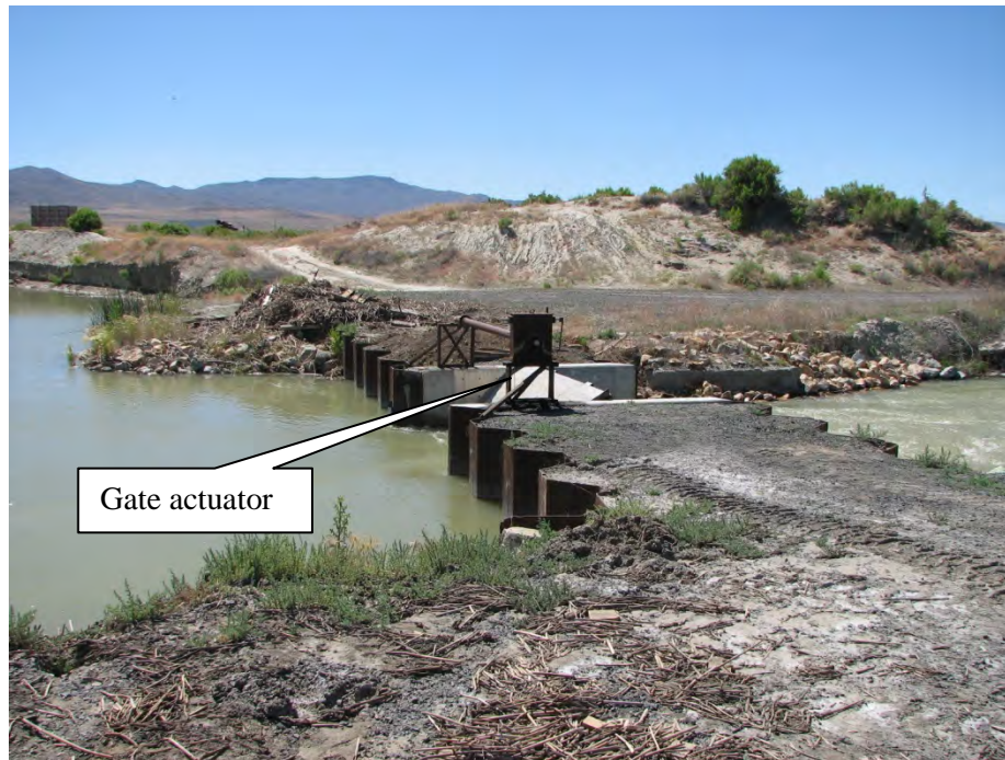
Figure 9 – Rogers Diversion Structure and existing gate actuator
