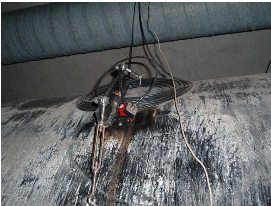
Figure 2 – Example of external flow sensor on penstock pipe
