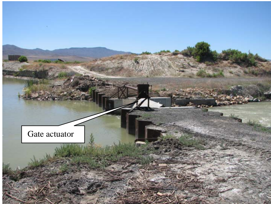
Figure 9 – Rogers Diversion Structure and existing gate actuator
