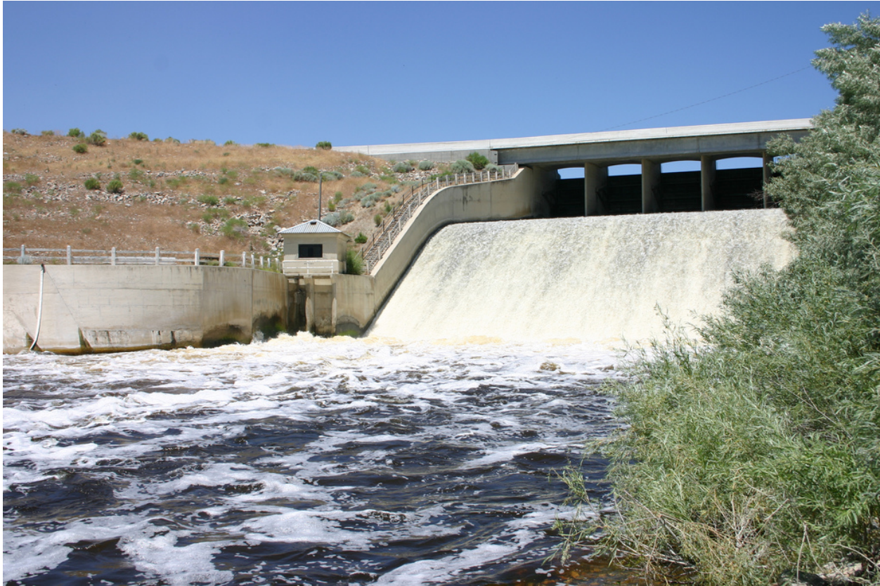
Figure 6 - Rye Patch Dam spillway and gate house
