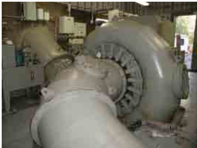
Volta 2 Powerhouse—Hydroelectric Turbine
