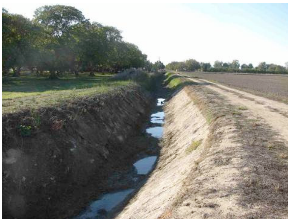
Photo 4. Main Canal north of Highway 20, facing north, November 7, 2011. Canal is lined in this area, but there are some areas of cracking and missing concrete.
