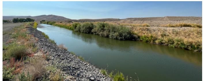
*The Truckee Canal's highest risk area is in the City of Fernley where 3.5 miles of the Canal will be reinforced and the Fernley Check Structure replaced.*
