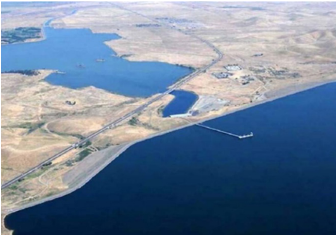
B.F. Sisk Dam is 3.5-miles long; it impounds San Luis Reservoir that provides water to communities, farmland, and Pacific Flyway wetlands south-of-the-Delta.
