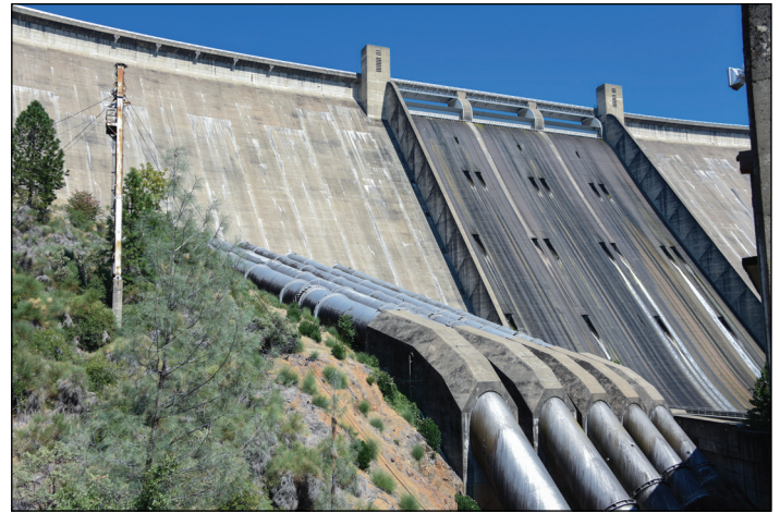
Shasta Powerplant sits beneath the dam and receives water via five penstocks.
