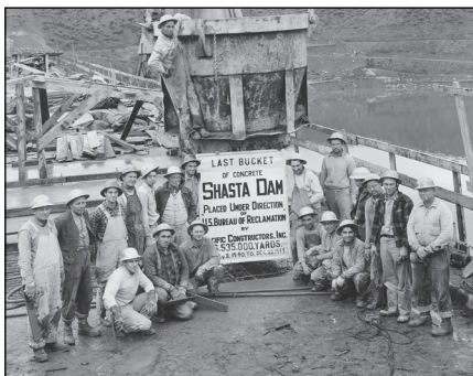
The last bucket of concrete placed to construct Shasta Dam
