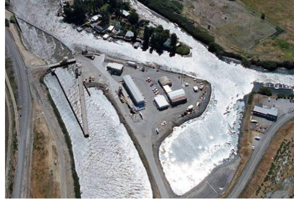
Aerial view of the Tracy Fish Collection Facility
