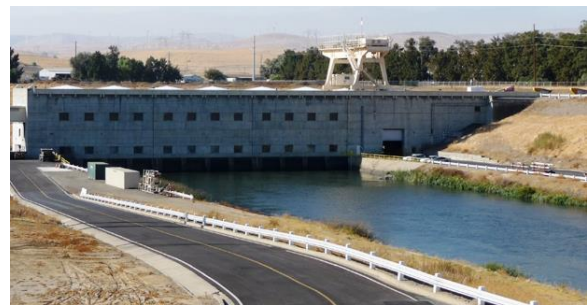
The C.W "Bill" Jones Pumping Plant
