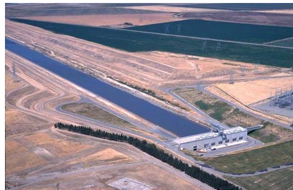
The Delta-Mendota Canal flows from the pumping plant
