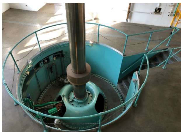
Shown is one of the plant's six motors, all of which recently underwent a successful rewind maintenance project, funded by Reclamation.
