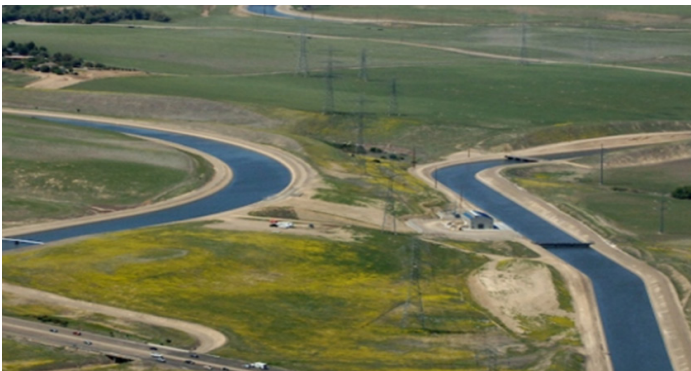
The 500-foot-long Intertie connects the California Aqueduct on the left to the Delta-Mendota Canal on the right.
