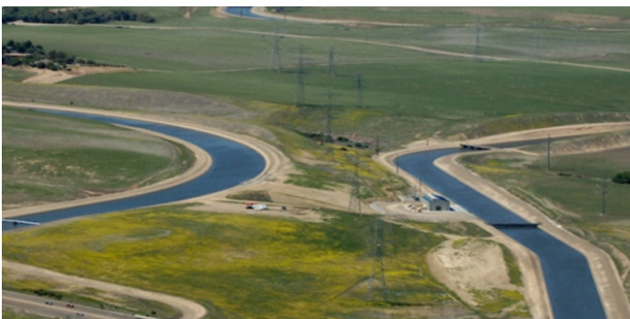
The 500-foot-long Intertie connects the California Aqueduct on the left to the Delta-Mendota Canal on the right.
