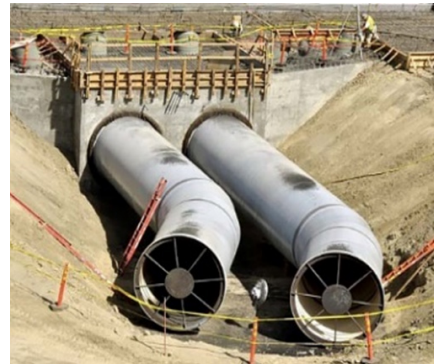
Intertie is shown while under construction.
