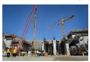
After excavating more than 2.5 million cubic yards of rock and soil for the spillway site, Reclamation handed the project over to the Corps' Sacramento District in January 2011. The Corps eventually removed more than 315,000 cubic yards of earth and constructed the approach channel, control structure, concrete-lined spillway chute, and stilling basin. The spillway was ready for use in fall 2017.
