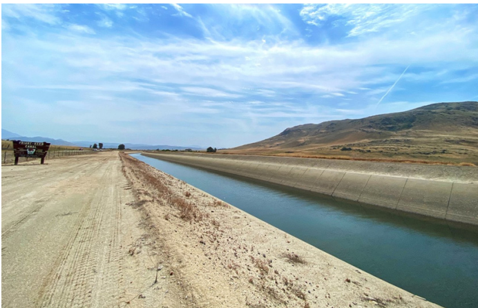
The Friant-Kern Canal near Fresno.
