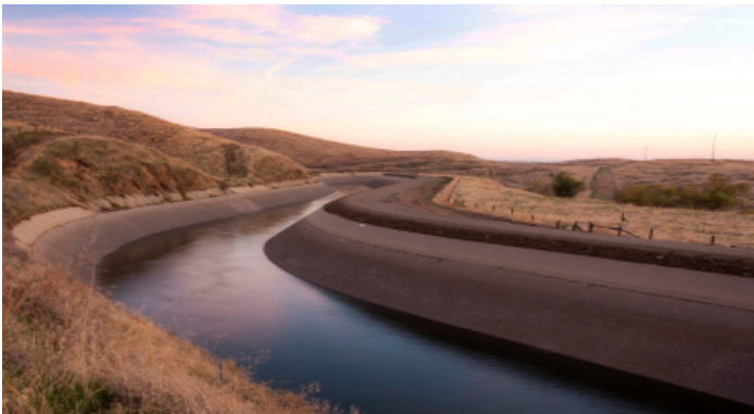
The Friant-Kern Canal
