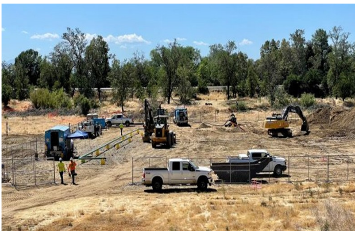
The Project site excavation includes removing around 90,500 cubic yards of material from about 20 acres at river mile 246 near Red Bluff.
