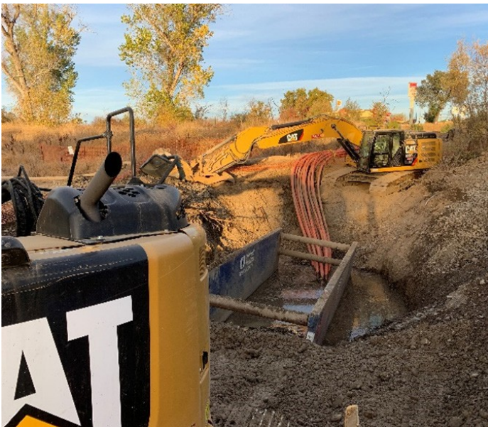
The excavator is relocating utility lines for telecommunications.
