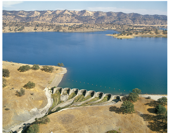
The 2,000-foot-long East Park Dam Spillway features a set of curved labyrinth-spillway fins.
