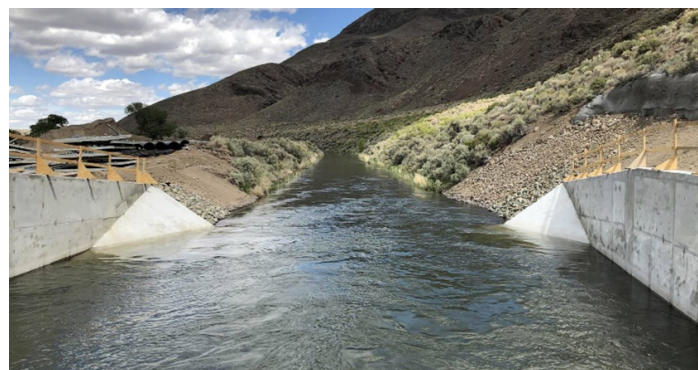
The end of the project where the new concrete afterbay transitions to the Truckee Canal.
