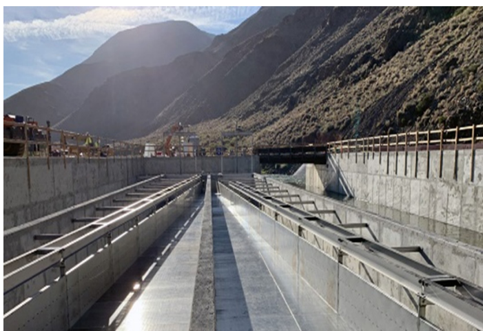
The horizontal fish screen at Derby Dam is the largest of its kind and allows fish to safely pass around Derby Dam.
